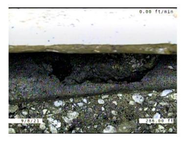
Code: SMW Description: Surface Damage Missing Wall Distance (ft): 286.0 Structural Grade: 5 O&M Grade: 0 Clock Start/From: 11 12 Clock To: 1st Value: 2nd Value:
