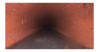
Code: MMC Description: **Material Change** Distance (ft): 115.6 Structural Grade: 0 O&M Grade: 0 Clock Start/From: Clock To: 1st Value: 2nd Value: Value Percent: Continuous Index: Within 8" of Joint: NO Remarks: VCP
