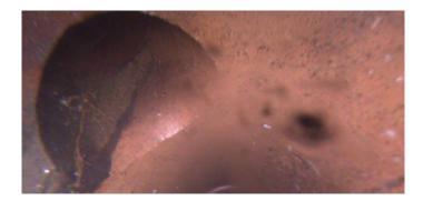
Code: TFD **Tap Factory Defective** Description: Distance (ft): 43.8 Structural Grade: 0 O&M Grade: 2 Clock Start/From: 11 Clock To: 1st Value: 4.000 2nd Value: Value Percent: Continuous Index: Within 8" of Joint: Remarks: rfl
