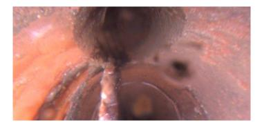
Code: TFD **Tap Factory Defective** Description: 57.8 Distance (ft): Structural Grade: 0 O&M Grade: 2 Clock Start/From: 12 Clock To: 1st Value: 4.000 2nd Value: Value Percent: Continuous Index: Within 8" of Joint: Remarks: ROOTS
