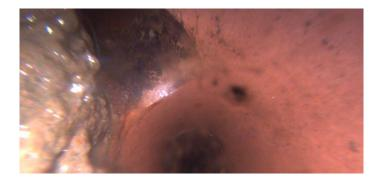
Code: TFD **Tap Factory Defective** Description: Distance (ft): 111.5 Structural Grade: 0 O&M Grade: 2 Clock Start/From: 11 Clock To: 1st Value: 4.000 2nd Value: Value Percent:
