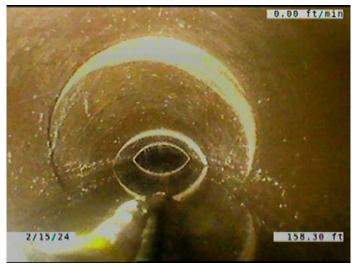
Code: MGO Description: **Miscellaneous General Observation** Distance (ft): 158.3 Structural Grade: 0 0 O&M Grade: Clock Start/From: Clock To: 1st Value: 2nd Value: Value Percent: Continuous Index: Within 8" of Joint: NO Remarks: A VIEW OF THE SAG FROM THE BACK UP CAMERA.
