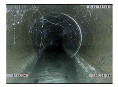
Code: MWLS Description: **Miscellaneous Water Level Sag** Distance (ft): 105.3 Structural Grade: 4 O&M Grade: 0 Clock Start/From: Clock To: 1st Value: 2nd Value: 55.000 Value Percent: Continuous Index: S08 Within 8" of Joint: NO Remarks:
