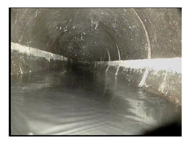
Code: MSA Description: Abandoned Survey Distance (ft): 110.0 Structural Grade: 0 O&M Grade: 0 Clock Start/From: Clock To: 1st Value: 2nd Value: Value Percent: Continuous Index: Within 8" of Joint: NO Remarks: sediment
