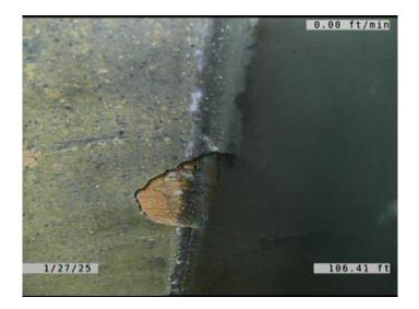
Code: Description: SSS Surface Damage Surface Spalling
