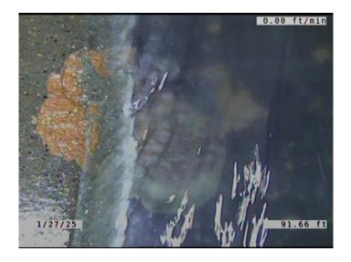
Code:SSCDescription:Surface Spalling of Damage Coating
