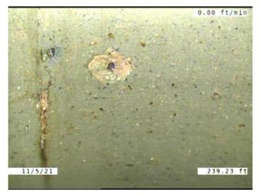
Code: SSS Description: Surface Damage Surface Spalling Distance (ft): 239.2 Structural Grade: 2 O&M Grade: 0 Clock Start/From: 10 Clock To: 1st Value: 2nd Value: Value Percent: Continuous Index: Within 8" of Joint: NO
