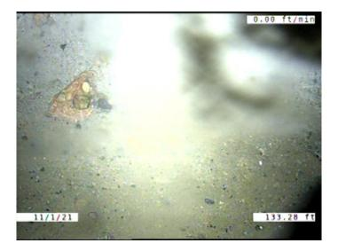
Code: SSS Description: Surface Damage Surface Spalling Distance (ft): 133.3 Structural Grade: 2 O&M Grade: 0 Clock Start/From: 1 Clock To: 1st Value: 2nd Value: Value Percent: Continuous Index: Within 8" of Joint: NO
