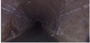
Distance (ft): 154.8 Structural Grade: 0 O&M Grade: 2 Clock Start/From: 8 9 Clock To: 1st Value: 2nd Value: Value Percent: Continuous Index: Within 8" of Joint: YES
