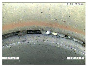
Code: JOMD Description: Joint Offset Medium Defective Distance (ft): 136.0 Structural Grade: 3 O&M Grade: 0 Clock Start/From: Clock To: 1st Value: 2nd Value: Value Percent: Continuous Index: Within 8" of Joint: NO Remarks:
