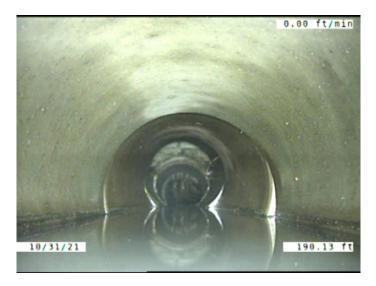
Code: MWLS Description: **Miscellaneous Water Level Sag** Distance (ft): 190.1 Structural Grade: 2 O&M Grade: 0 Clock Start/From: Clock To: 1st Value: 2nd Value: Value Percent: 15.000 Continuous Index: Within 8" of Joint: NO Remarks:
