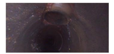
Distance (ft): 12.9 Structural Grade: 0 O&M Grade: 0 Clock Start/From: 1
