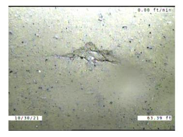
Code: SSS Description: Surface Damage Surface Spalling 63.4 Distance (ft): Structural Grade: 2 O&M Grade: 0 Clock Start/From: 2 Clock To: 1st Value: 2nd Value: Value Percent: Continuous Index: Within 8" of Joint: YES
