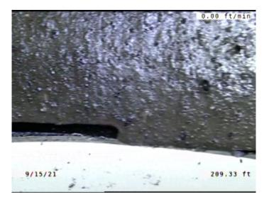
Code: MMC Description: **Miscellaneous Material Change** Distance (ft): 209.3 Structural Grade: 0 O&M Grade: 0 Clock Start/From: Clock To: 1st Value: 2nd Value: Value Percent: Continuous Index: Within 8" of Joint: NO VCP TO PVC Remarks:
