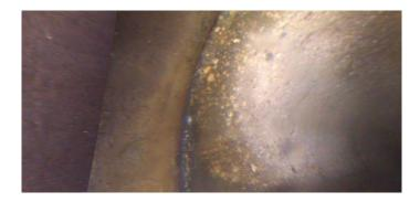
Code: MMC Description: **Material Change** Distance (ft): 167.1 Structural Grade: 0 O&M Grade: 0 Clock Start/From: Clock To: 1st Value: 2nd Value: Value Percent: Continuous Index: Within 8" of Joint: NO Remarks: vcp
