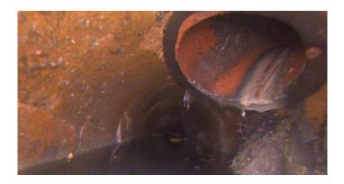
Code: TBD Description: **Tap Break-in Defective** Distance (ft): 39.0 Structural Grade: 0 O&M Grade: 3 Clock Start/From: 2 Clock To: 1st Value: 4.000 2nd Value: Value Percent: Continuous Index:
