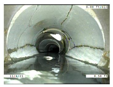
Code: Description: **Broken** Distance (ft): .5 Structural Grade: 4 0 O&M Grade: Clock Start/From: 8 Clock To: 4 1st Value: 2nd Value: Value Percent:
