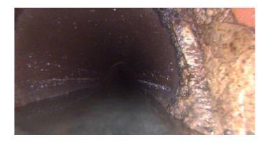
Code: DAZ Description: **Deposits Attached Other** Distance (ft): 19.9 Structural Grade: 0 O&M Grade: 2 Clock Start/From: 7 Clock To: 5 1st Value: 2nd Value: Value Percent: 5.000 Continuous Index:
