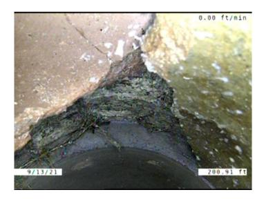
Distance (ft): 200.9 Structural Grade: 4 O&M Grade: 0 Clock Start/From: 10 Clock To: 2 1st Value: 2nd Value: Value Percent: Continuous Index: Within 8" of Joint: YES
