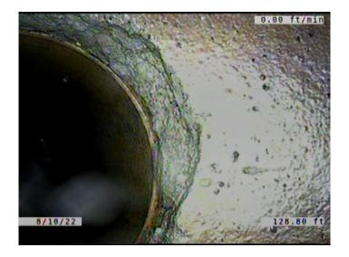
Code:SSSDescription:Surface Damage Surface SpallingDistance (ft):128.8Structural Grade:2
