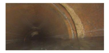
Code: Description: CL Crack Longitudinal
