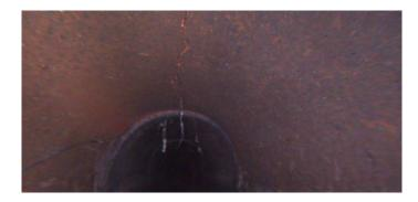
Code: FM Description: **Fracture Multiple** Distance (ft): 5.7 Structural Grade: 4 O&M Grade: 0 Clock Start/From: 8 Clock To: 12 1st Value: 2nd Value: Value Percent: Continuous Index: S01 Within 8" of Joint: YES Remarks: wandering
