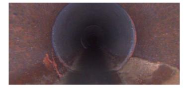
Distance (ft): .0 Structural Grade: 4 O&M Grade: 0 Clock Start/From: 7 Clock To: 5 1st Value: 2nd Value: Value Percent: Continuous Index: **S01** Within 8" of Joint: YES
