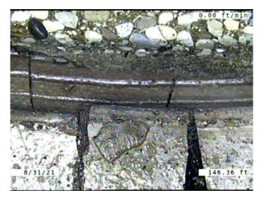
Code: MMC Description: **Miscellaneous Material Change** Distance (ft): 146.4 Structural Grade: 0 O&M Grade: 0 Clock Start/From: Clock To: 1st Value: 2nd Value: Value Percent: Continuous Index: Within 8" of Joint: NO Remarks: CONCRETE TO VCP
