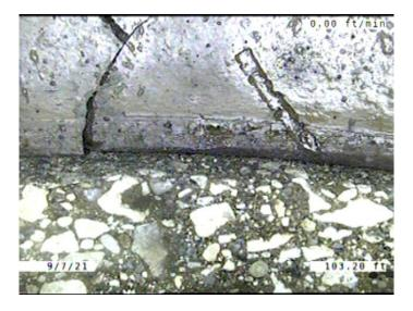
Code: MMC Description: **Miscellaneous Material Change** Distance (ft): 103.2 Structural Grade: 0 O&M Grade: 0 Clock Start/From: Clock To: 1st Value: 2nd Value: Value Percent: Continuous Index: Within 8" of Joint: NO Remarks: **VCP TO CONCRETE**
