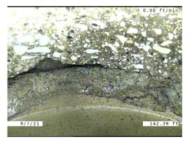
Code: MMC Description: **Miscellaneous Material Change** Distance (ft): 142.4 Structural Grade: 0 O&M Grade: 0 Clock Start/From: Clock To: 1st Value: 2nd Value: Value Percent: Continuous Index: Within 8" of Joint: NO Remarks: CONCRETE TO VCP
