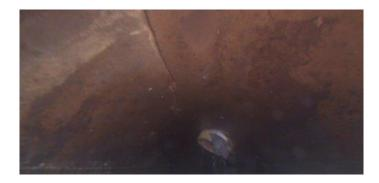
Code: MMC Description: **Material Change** Distance (ft): 16.1 Structural Grade: 0 O&M Grade: 0 Clock Start/From: Clock To: 1st Value: 2nd Value: Value Percent: Continuous Index: Within 8" of Joint: NO
