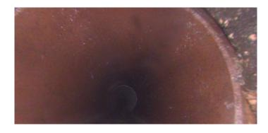
Code: MMC Description: **Material Change** Distance (ft): 119.2 Structural Grade: 0 O&M Grade: 0 Clock Start/From: Clock To: 1st Value: 2nd Value: Value Percent: Continuous Index: Within 8" of Joint: NO
