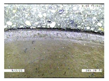
Code: MMC Description: **Miscellaneous Material Change** Distance (ft): 205.7 Structural Grade: 0 O&M Grade: 0 Clock Start/From: Clock To: 1st Value: 2nd Value: Value Percent: Continuous Index: Within 8" of Joint: NO Remarks: CONCRETE TO VCP
