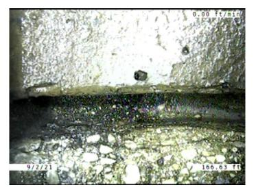
Code: MMC Description: **Miscellaneous Material Change** Distance (ft): 166.6 Structural Grade: 0 O&M Grade: 0 Clock Start/From: Clock To: 1st Value: 2nd Value: Value Percent: Continuous Index: Within 8" of Joint: NO Remarks: **VCP TO CONCRETE**
