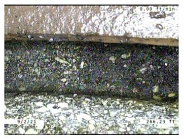
Code: MMC Description: **Miscellaneous Material Change** Distance (ft): 266.2 Structural Grade: 0 O&M Grade: 0 Clock Start/From: Clock To: 1st Value: 2nd Value: Value Percent: Continuous Index: Within 8" of Joint: NO Remarks: **VCP TO CONCRETE**
