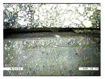
Code: MMC Description: **Miscellaneous Material Change** Distance (ft): 160.7 Structural Grade: 0 O&M Grade: 0 Clock Start/From: Clock To: 1st Value: 2nd Value: Value Percent: Continuous Index: Within 8" of Joint: NO Remarks: CONCRETE TO VCP
