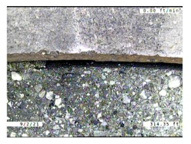
Code: MMC Description: **Miscellaneous Material Change** Distance (ft): 314.4 Structural Grade: 0 0 O&M Grade: Clock Start/From: Clock To: 1st Value: 2nd Value: Value Percent: Continuous Index: Within 8" of Joint: NO Remarks: **VCP TO CONCRETE**
