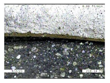
Code: MMC Description: **Miscellaneous Material Change** Distance (ft): 210.1 Structural Grade: 0 O&M Grade: 0 Clock Start/From: Clock To: 1st Value: 2nd Value: Value Percent: Continuous Index: Within 8" of Joint: NO Remarks: VCP TO CONCRETE
