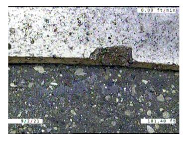
Code: MMC Description: **Miscellaneous Material Change** Distance (ft): 101.4 Structural Grade: 0 O&M Grade: 0 Clock Start/From: Clock To: 1st Value: 2nd Value: Value Percent: Continuous Index: Within 8" of Joint: NO Remarks: **VCP TO CONCRETE**
