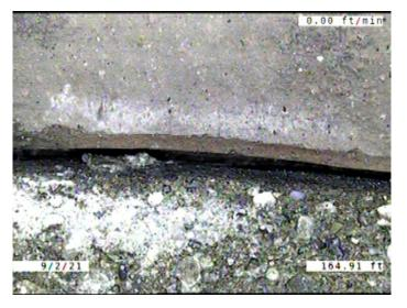
Code: MMC Description: **Miscellaneous Material Change** Distance (ft): 164.9 Structural Grade: 0 0 O&M Grade: Clock Start/From: Clock To: 1st Value: 2nd Value: Value Percent: Continuous Index: Within 8" of Joint: NO Remarks: **VCP TO CONCRETE**
