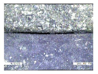
Code: MMC Description: **Miscellaneous Material Change** Distance (ft): 161.8 Structural Grade: 0 O&M Grade: 0 Clock Start/From: Clock To: 1st Value: 2nd Value: Value Percent: Continuous Index: Within 8" of Joint: NO Remarks: CONCRETE TO VCP
