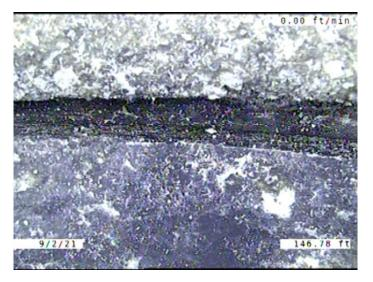
Code: MMC Description: **Miscellaneous Material Change** Distance (ft): 146.8 Structural Grade: 0 O&M Grade: 0 Clock Start/From: Clock To: 1st Value: 2nd Value: Value Percent: Continuous Index: Within 8" of Joint: NO Remarks: CONCRETE TO VCP
