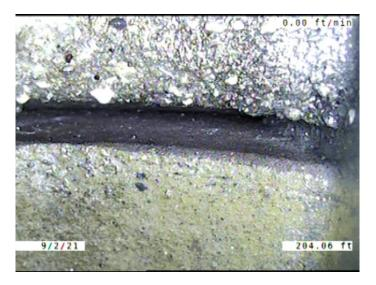
Code: MMC Description: **Miscellaneous Material Change** Distance (ft): 204.1 Structural Grade: 0 O&M Grade: 0 Clock Start/From: Clock To: 1st Value: 2nd Value: Value Percent: Continuous Index: Within 8" of Joint: NO Remarks: CONCRETE TO VCP
