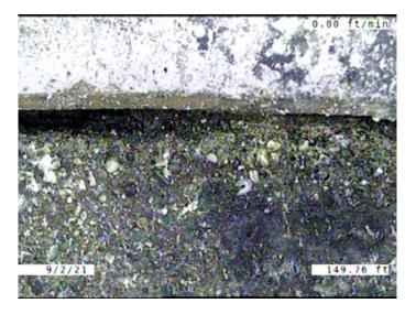
Code: MMC Description: **Miscellaneous Material Change** Distance (ft): 149.8 Structural Grade: 0 O&M Grade: 0 Clock Start/From: Clock To: 1st Value: 2nd Value: Value Percent: Continuous Index: Within 8" of Joint: NO Remarks: **VCP TO CONCRETE**
