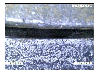
Code: JSL Description: Joint Separated Large Distance (ft): 135.6 Structural Grade: 4 O&M Grade: 0 Clock Start/From: Clock To: 1st Value: 2nd Value: Value Percent: Continuous Index: Within 8" of Joint: NO Remarks: SOIL VISIBLE
