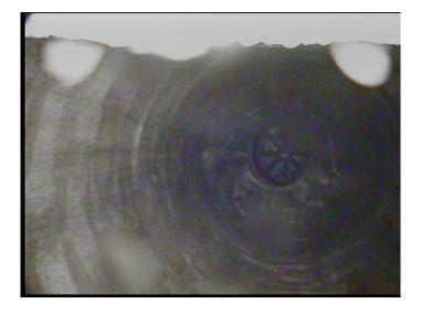
Code: SAV Description: Surface Aggregate Visible Distance (ft): 310.9 Structural Grade: 3 O&M Grade: 0 Clock Start/From: 8 Clock To: 4 1st Value: 2nd Value: Value Percent: Continuous Index: F01 Within 8" of Joint: NO
