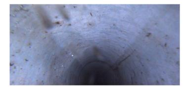
Code: LFAC Description: Lining Failure Abandoned Connection 22.4 Distance (ft): Structural Grade: 0 O&M Grade: 0 Clock Start/From: 10 Clock To: 1st Value: 2nd Value: Value Percent: Continuous Index: Within 8" of Joint: NO
