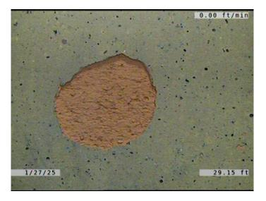
Code: SSC Description: Surface Spalling of Damage Coating Distance (ft): 29.2 Structural Grade: 1 O&M Grade: 0 Clock Start/From: 12 Clock To: 1st Value: 2nd Value: Value Percent: Continuous Index: Within 8" of Joint:
