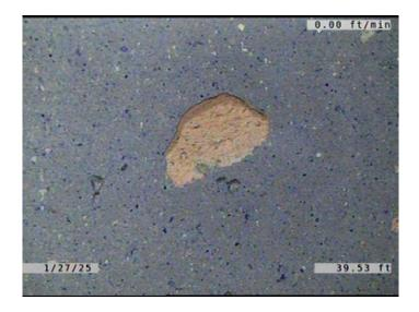
Code: SSC Description: Surface Spalling of Damage Coating Distance (ft): 39.5 Structural Grade: 1 O&M Grade: 0 Clock Start/From: 2 Clock To: 1st Value: 2nd Value: Value Percent: Continuous Index:
