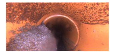
Code: RMJ Description: **Roots Medium Joint** 72.1 Distance (ft): Structural Grade: 0 O&M Grade: 3 Clock Start/From: 6 Clock To: 9 1st Value: 2nd Value: Value Percent: 40.000
