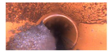
Code: RMJ Description: **Roots Medium Joint** 72.1 Distance (ft): Structural Grade: 0 O&M Grade: 3 Clock Start/From: 6 Clock To: 9 1st Value: 2nd Value:
