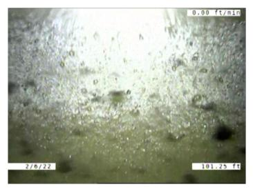
Code: MCU Description: Miscellaneous Camera Underwater Distance (ft): 101.3 Structural Grade: 0 O&M Grade: 4 Clock Start/From: Clock To: 1st Value: 2nd Value: Value Percent: Continuous Index: Within 8" of Joint: NO Remarks: Out at 102.6
