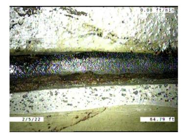
Code: JAM Description: Joint Angular Medium Distance (ft): 64.8 Structural Grade: 3 O&M Grade: 0 Clock Start/From: Clock To: 1st Value: 2nd Value: Value Percent: Continuous Index: Within 8" of Joint: NO Remarks:
