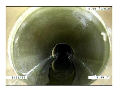
LD Code: Description: **Line Down** Distance (ft): 4.4 Structural Grade: 0 O&M Grade: 1 Clock Start/From: Clock To: 1st Value: 2nd Value: Value Percent: 5.000 Continuous Index: Within 8" of Joint: NO
