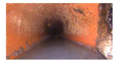
Code: DAZ Description: **Deposits Attached Other** Distance (ft): 65.9 Structural Grade: 0 O&M Grade: 2 Clock Start/From: 4 Clock To: 5 1st Value: 2nd Value: Value Percent: 5.000
