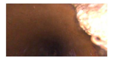
Code: DAGS Description: **Deposits Attached Grease** Distance (ft): 76.2 Structural Grade: 0 O&M Grade: 2 Clock Start/From: 2 4 Clock To: 1st Value: 2nd Value: 5.000 Value Percent: Continuous Index: Within 8" of Joint: YES
