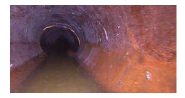
Code: Description: CL Crack Longitudinal
