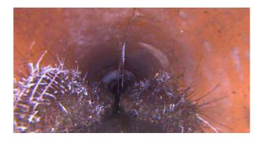
Code: RMB Description: **Roots Medium Barrel** Distance (ft): 151.3 Structural Grade: 0 O&M Grade: 4 Clock Start/From: 7 Clock To: 5 1st Value: 2nd Value: Value Percent: 10.000 Continuous Index:
