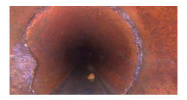
Code: RFJ Description: **Roots Fine Joint** Distance (ft): 30.9 Structural Grade: 0 O&M Grade: 1 Clock Start/From: 8 Clock To: 1st Value: 2nd Value: Value Percent: Continuous Index:
