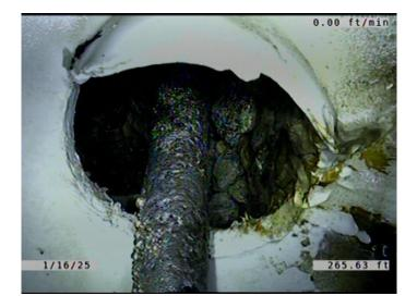
Code: IRB Description: Infiltration Runner Barrel Distance (ft): 265.6 Structural Grade: 0 O&M Grade: 4 Clock Start/From: 3 Clock To: 1st Value: 2nd Value: Value Percent: Continuous Index: Within 8" of Joint: YES Remarks:
