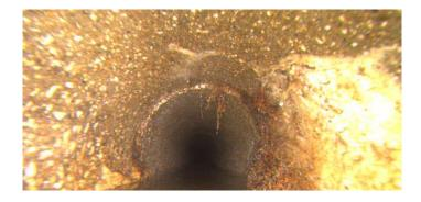
Code:FMDescription:Fracture MultipleDistance (ft):282.6Structural Grade:4O&M Grade:0Clock Start/From:8
