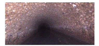
Distance (ft): 11.2 Structural Grade: 3 O&M Grade: 0 Clock Start/From: 8 Clock To: 4
