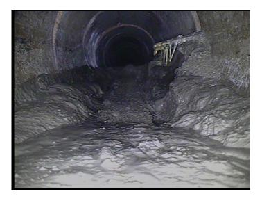
Code: MSA Description: Abandoned Survey Distance (ft): 118.5 Structural Grade: 0 O&M Grade: 0 Clock Start/From: Clock To: 1st Value: 2nd Value: Value Percent: Continuous Index: Within 8" of Joint: NO Remarks: heavy sediment
