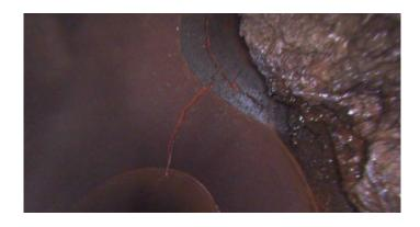
Code: TFD **Tap Factory Defective** Description: Distance (ft): 81.3 Structural Grade: 0 O&M Grade: 2 Clock Start/From: 2 Clock To: 1st Value: 4.000 2nd Value: Value Percent: Continuous Index: Within 8" of Joint: Remarks: Debris
