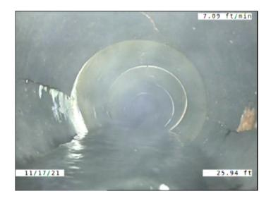
Description: Surface Damage Surface Spalling
