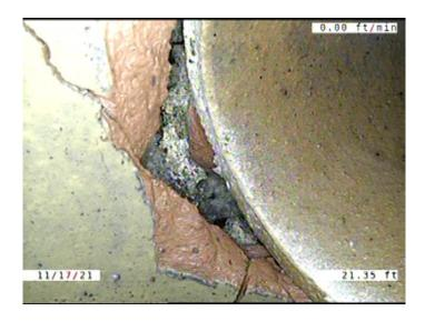
Description: **Surface Damage Surface Spalling**
