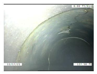
Code: Description: Broken Distance (ft): 8.6 Structural Grade: 4 0 O&M Grade: Clock Start/From: 12 Clock To: 12 1st Value: 2nd Value: Value Percent:
