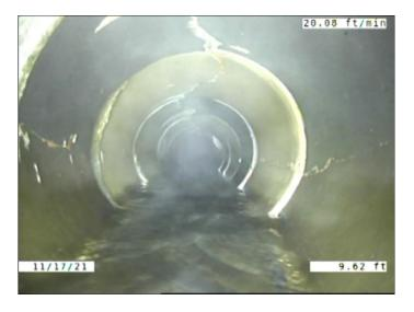
Code: FΜ Description: **Fracture Multiple** Distance (ft): 9.6 Structural Grade: 4 O&M Grade: 0 Clock Start/From: 8 Clock To: 4 1st Value: 2nd Value: Value Percent: Continuous Index: **S03** Within 8" of Joint: YES
