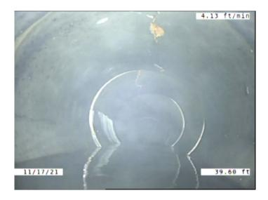
Description: **Surface Damage Surface Spalling**
