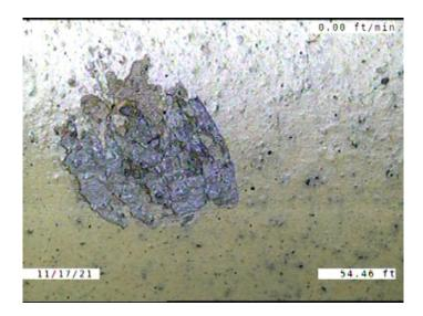
Description: **Surface Damage Surface Spalling**
